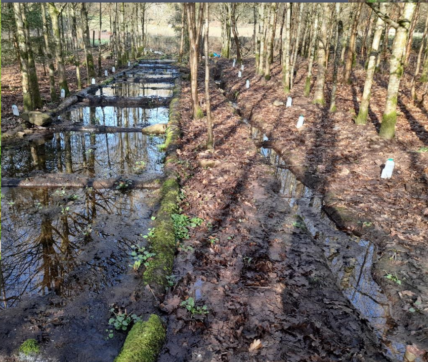
Cellular Runoff Attenuation Feature
