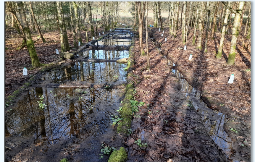
4. Runoff treatment swale
