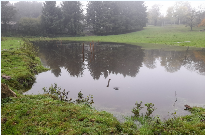
1. Flood detention basin
